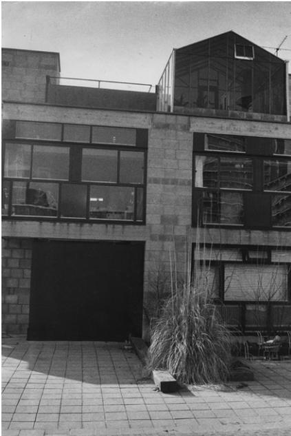
Window frames are designed in a way as to offer a choice of glass or rather closed panels. As long as it is filled in symmetrically it will always show a characteristic appearance. Probably this architectonic intervention, the way it literally wants to explain the idea of framework (structure) and infill, was pushing too far and did not really work out. Those windows that are not composed after this design principle are added by inhabitants in places of their own choice.
